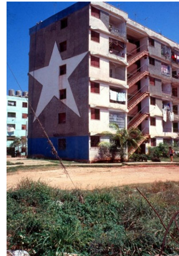
This block of apartment buildings was built by the Microbrigade systems, Alamar, 1970s. Photo: Roberto Segre.
