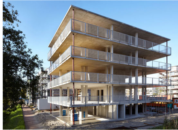
In the foundations and settlers model, residents build their own home within a concrete infrastructure provided by the architects Anne-Julchen Bernhardt and Jörg Leeser. Photo: Götz Wrage
