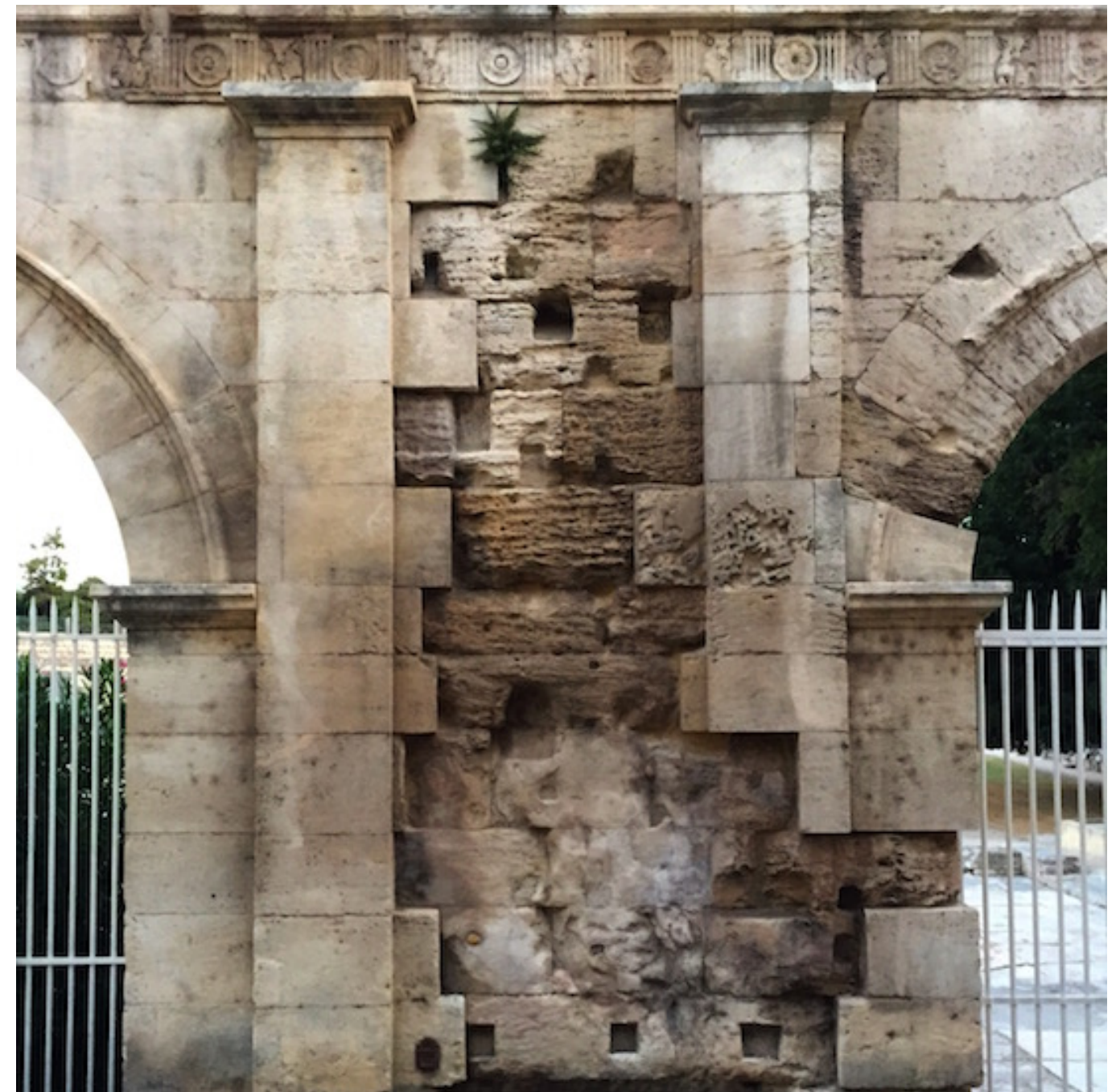
Limestone supplements frame the original stones of the ancient Roman theater in Arles, France. Photo: Jorge Otero-Pailos.
