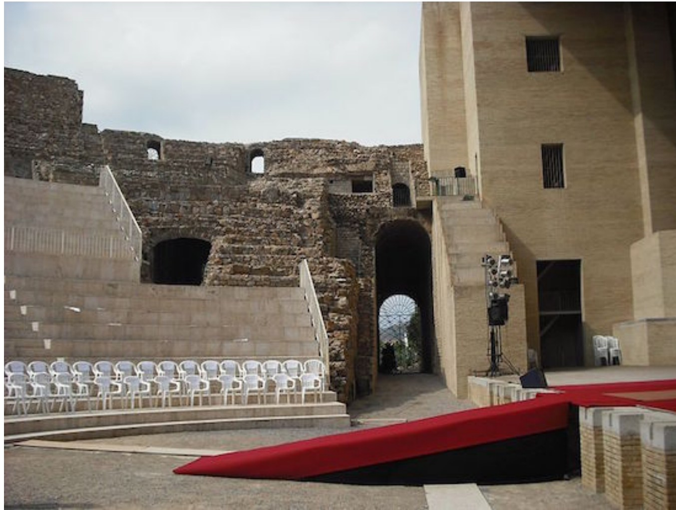
Supplemental brick scaenae frons and Tudela stone cavea seating frame the original stones of the Roman theater in Sagunto, Spain. The design by Giorgio Grassi and Manuel Portaceli was completed in 1993 and received with much criticism. Photo: Iniguez Rodriguez Enrique, Wikimedia Commons.
