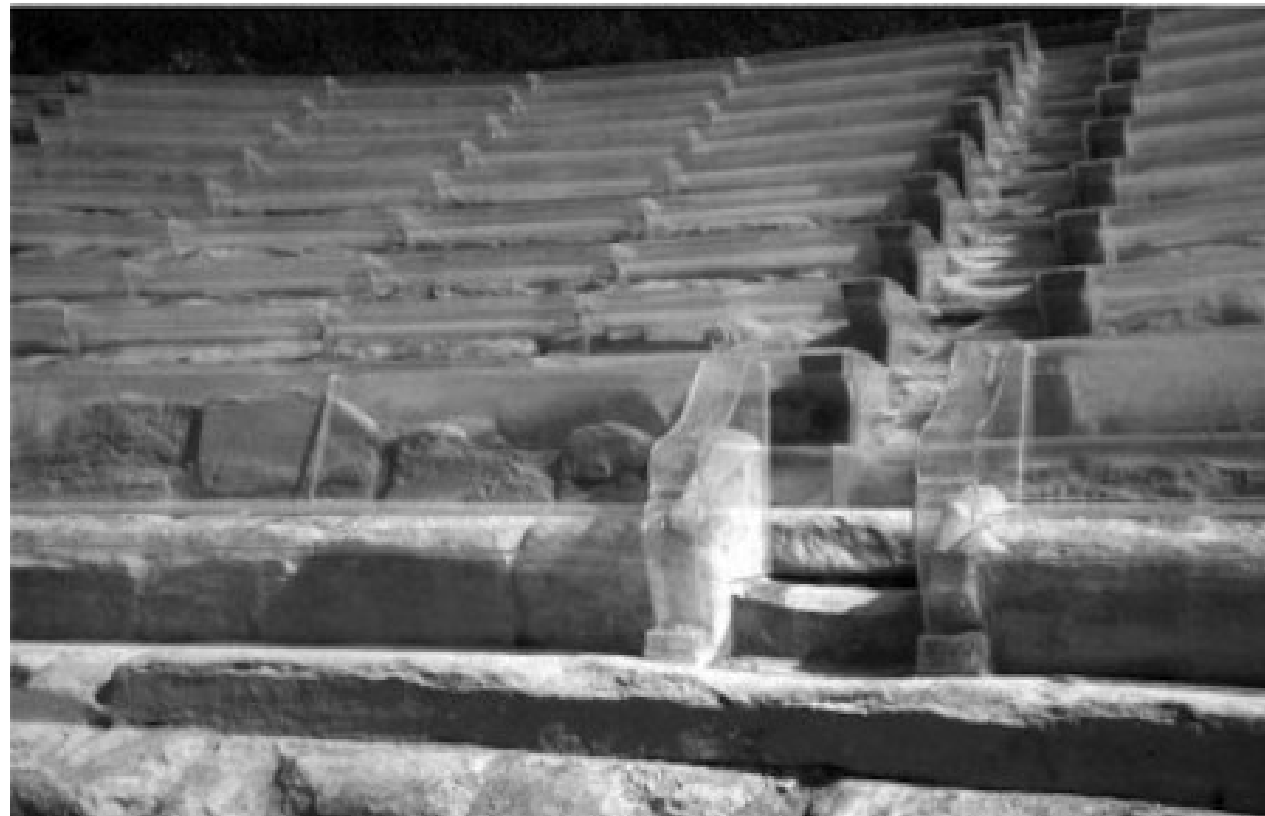
Supplemental plexiglass seating over the original stones of the Greek Theater at Heraclea Minoa, Agrigento, designed by Franco Minissi (1960–63). Left: as built in 1973. Photo courtesy of C. Bellanca. Right: The first level of bleachers with breaking laminate and greenery infestation, 2000, (N. P. Stanley-Price, J. Jokilehto, "The decision to shelter archaeological sites: Three case studies from Sicily," Conservation and Management of Archaeological Sites no. 5, 2001: 19–34).
